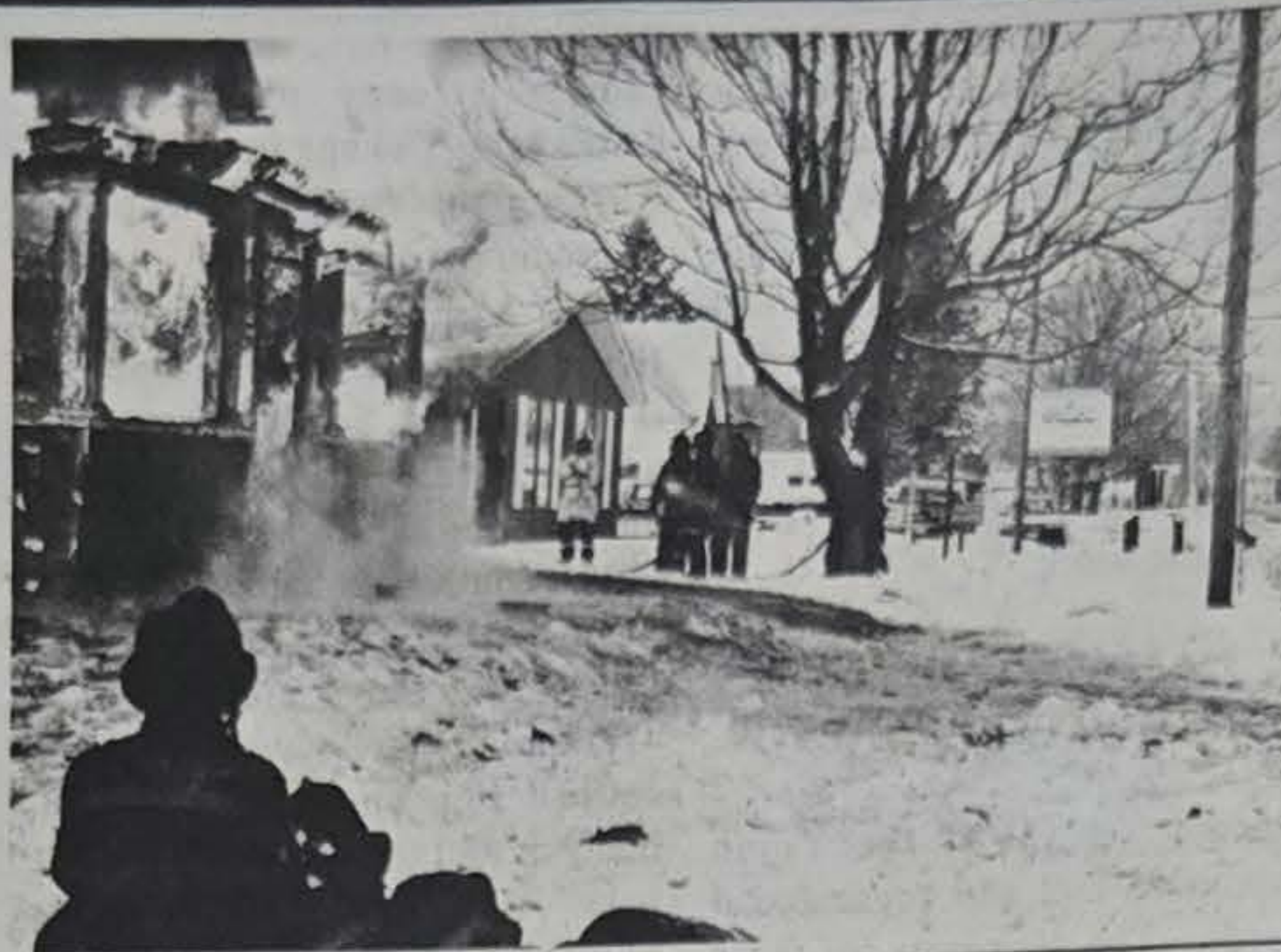
Good Bye to the Old and Welcome to the New The Fire Department and Dick Porter face many new challenges with the burn of this home.
