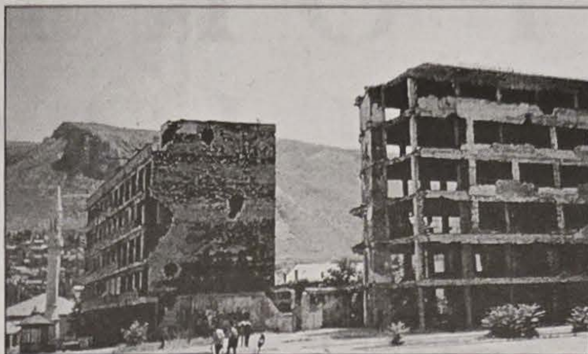
These bombed and shelled out office and apartment buildings were along the main line of fighting in Mostar. Scenes such as these are common in many of the areas Chief Hufford works in every day.
