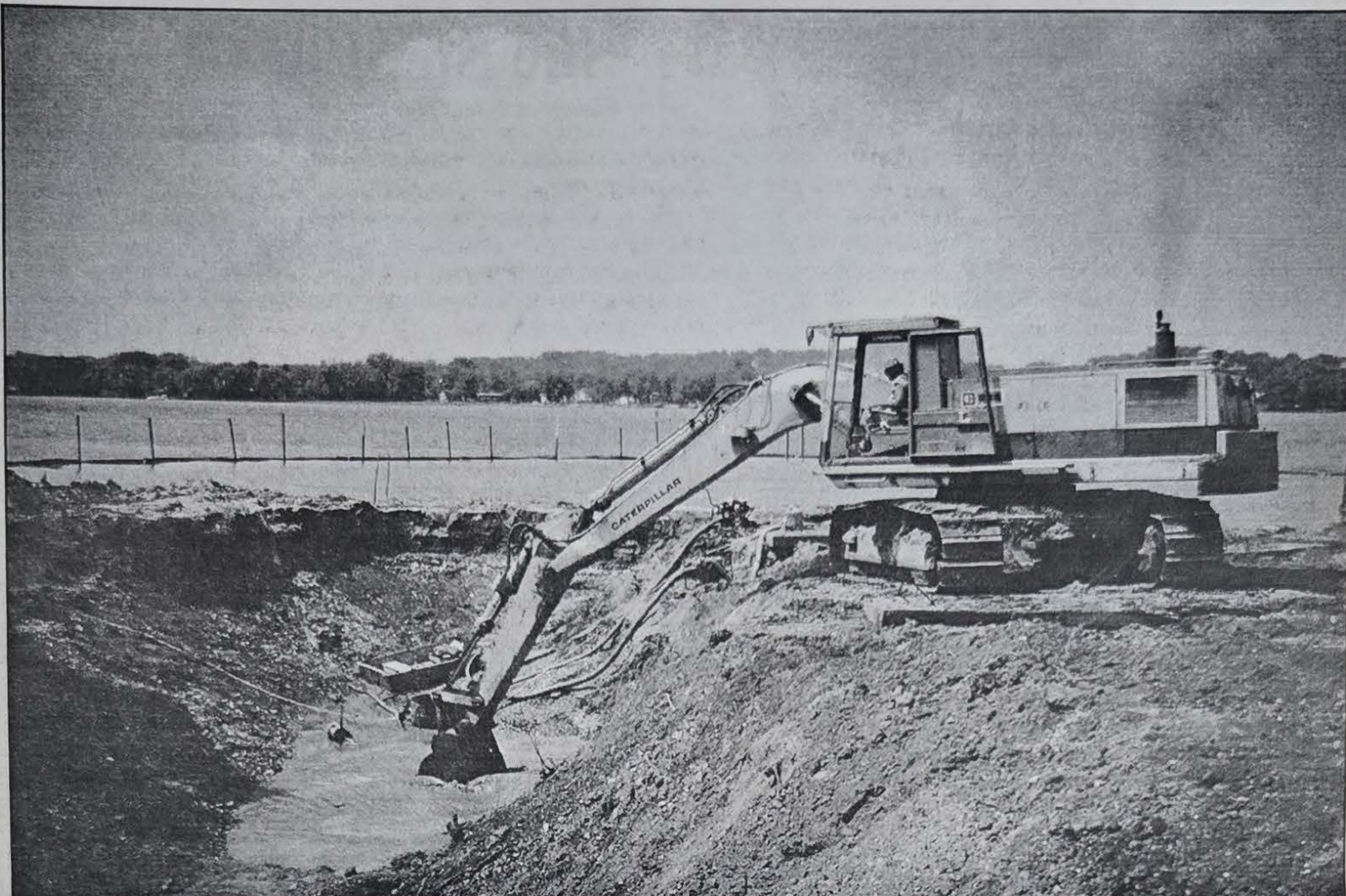
Hampton marina-condominium project is underway. Heartland Development/Twin Rivers Construction digs a nine foot deep channel from the quarry to the river. In the background, the line of posts holds a silt fence that holds 95% of any disturbed soil. Developer John McChurch projects many of the condos and dock slips will be sold this fall. The condos will sell from $250,000 to $400,000 with private boat slips going for $25,000 each. (Photo by Michaela VanDieren)
