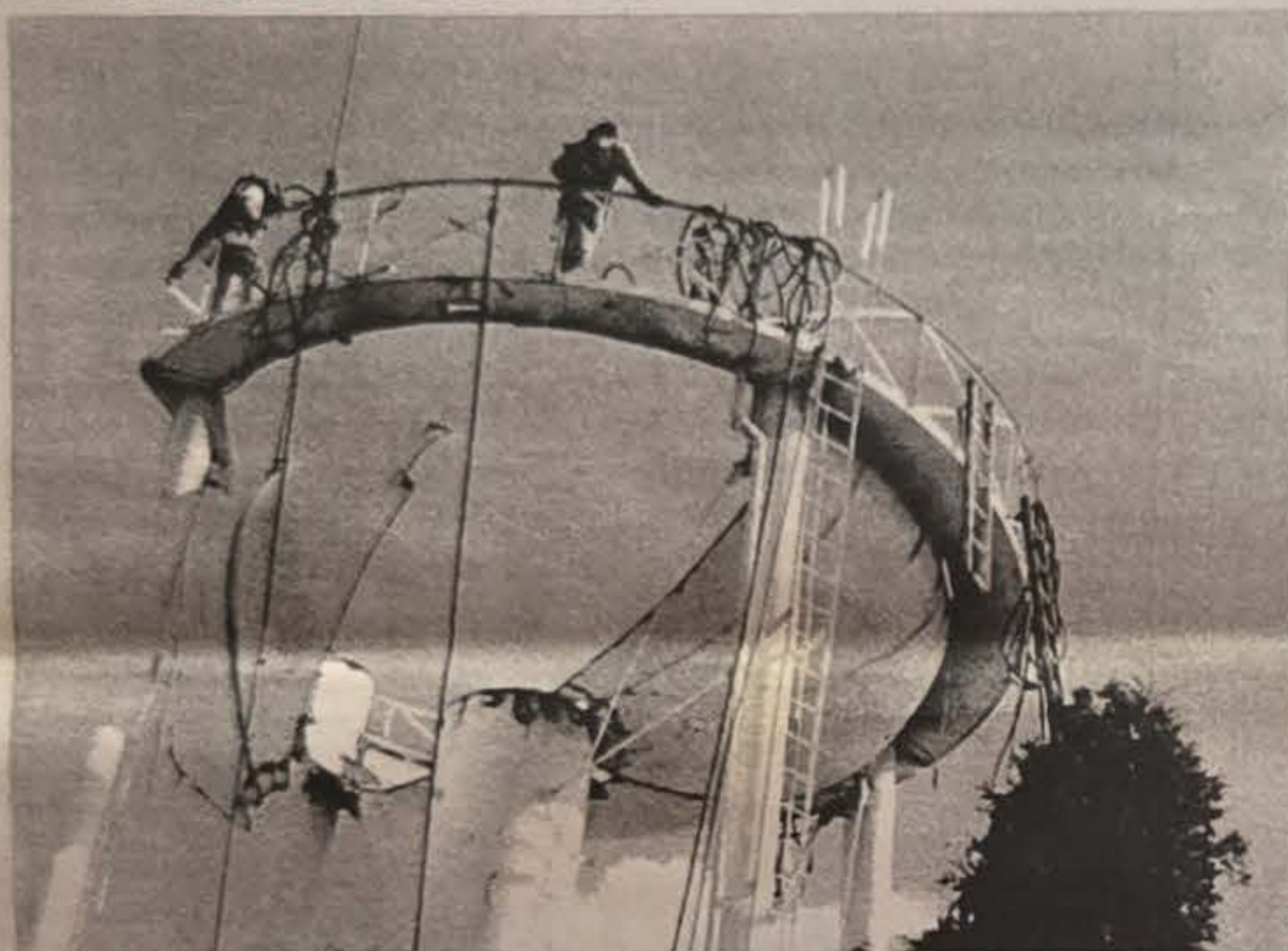
Little remains of the old water tower. Workers dismantled the tower in sections. (I wouldn't feel comfortable standing where they are working.)
