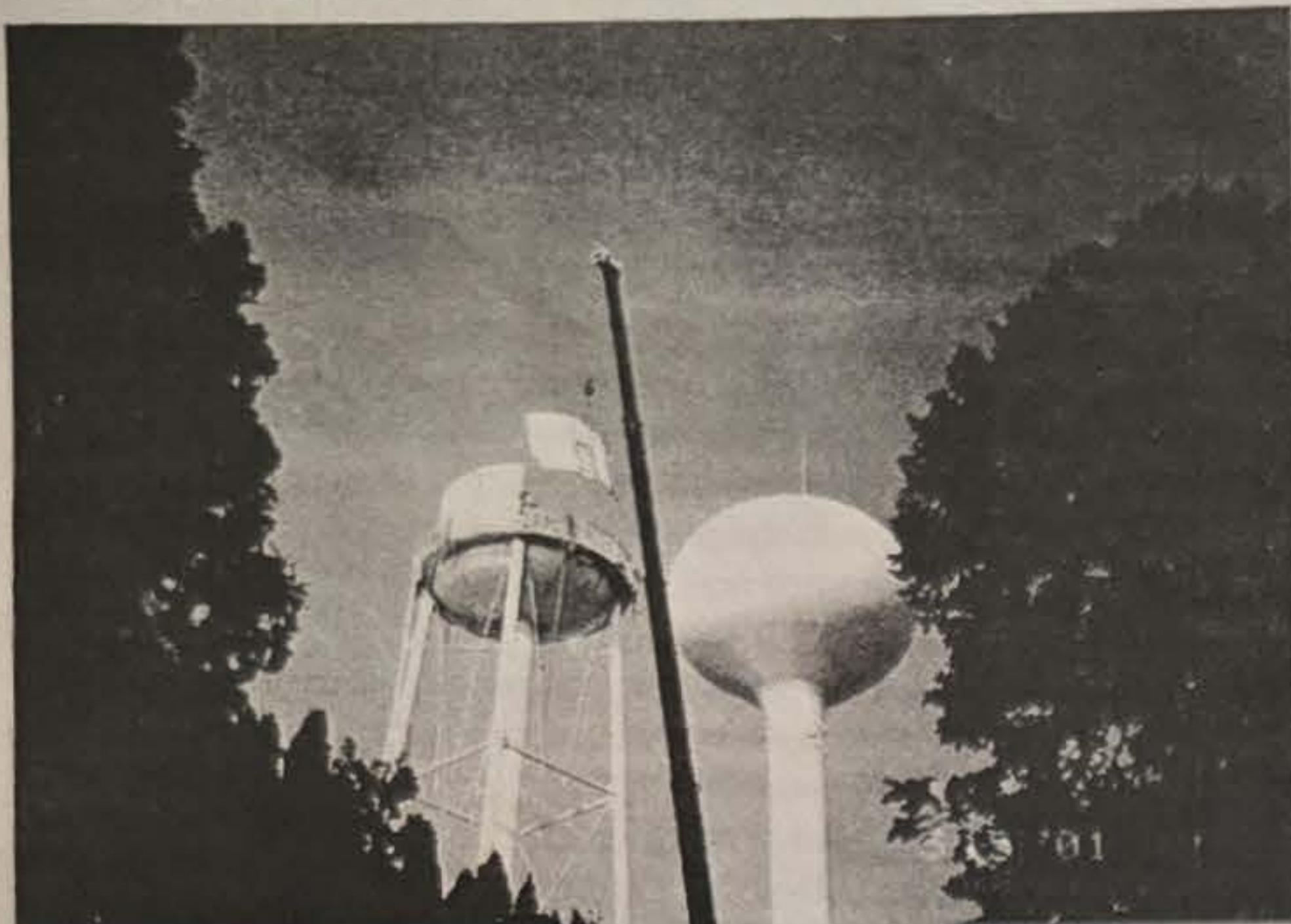
A crane carefully lowers a section of the old water tower with the new tower seen in the background.
