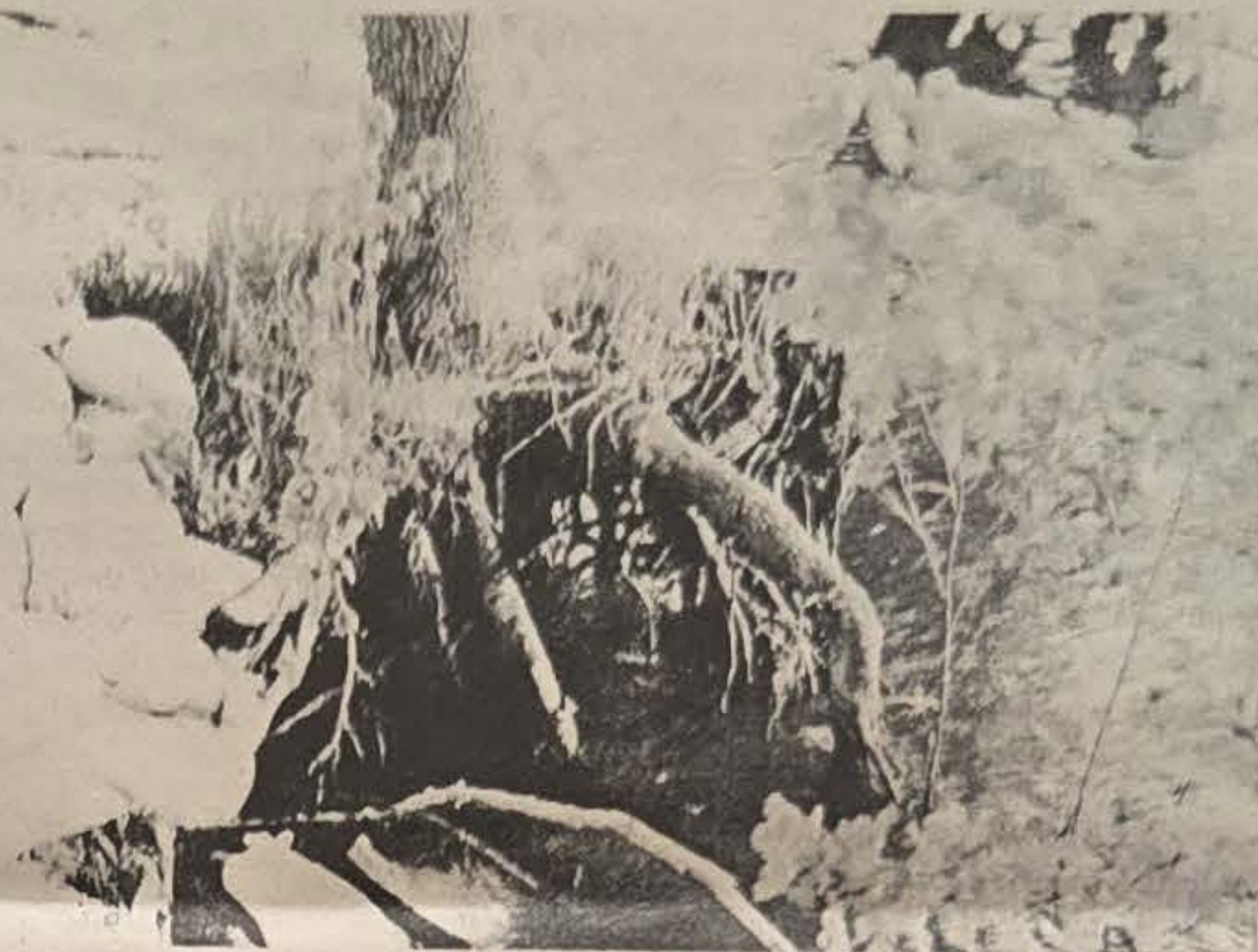
Roger Gunneman captured some of the washouts by the bike path in the Mississippi River Park. Volunteers sandbagged the banks to prevent further damage.
