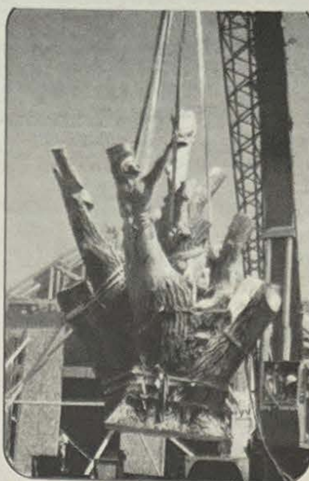
Steps 5 and 6: Lifting the tree from the truck with a crane, to put it into the Center through the roof.
