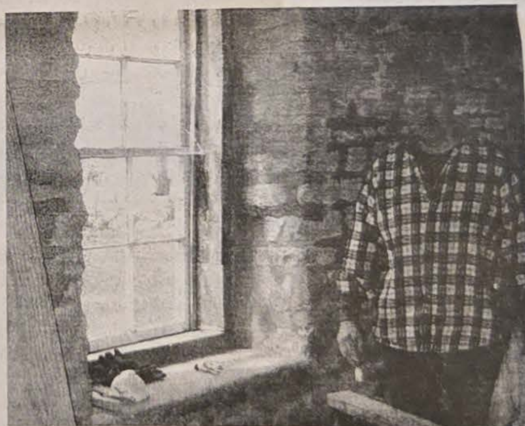
John Pischke, working in the lower level of the Brettun & Black Museum's limestone foundation.
