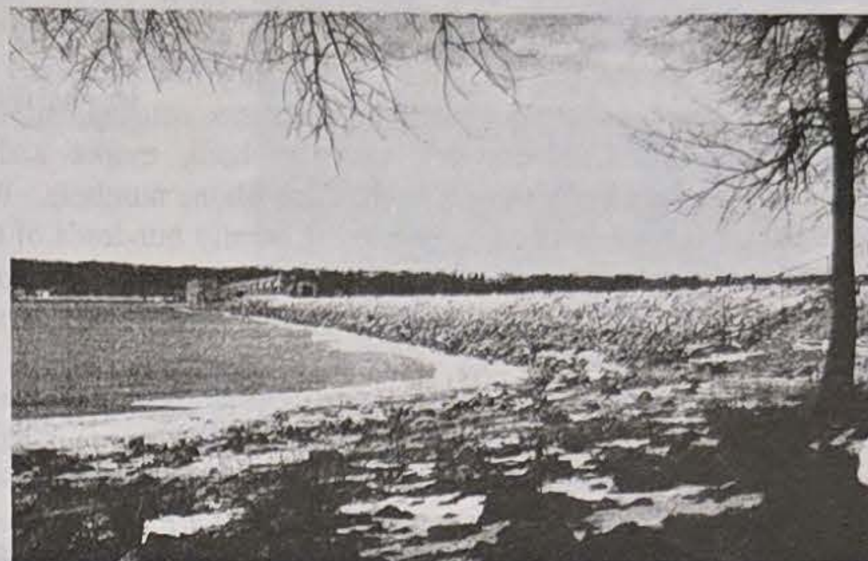
View of Lock and Dam #14 from Illinois side parking lot
