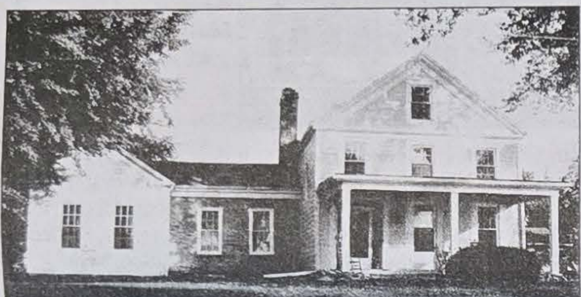
Located 500 Block of First Avenue
